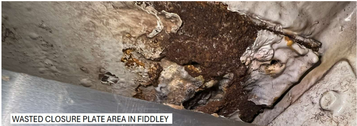
CLOSURE PLATE IN FIDDLEY WITH EXISTING SPLASHZONE PATCHES
